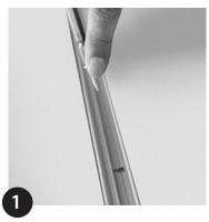
Drill holes for screws (2 per 500mm/20") and rear cable entry (10mm/0.39" min.) and coat raceway with corrosion inhibitor if required.
